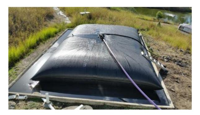
3. The water in the pump well is pumped back to the main holding tank at the STP
